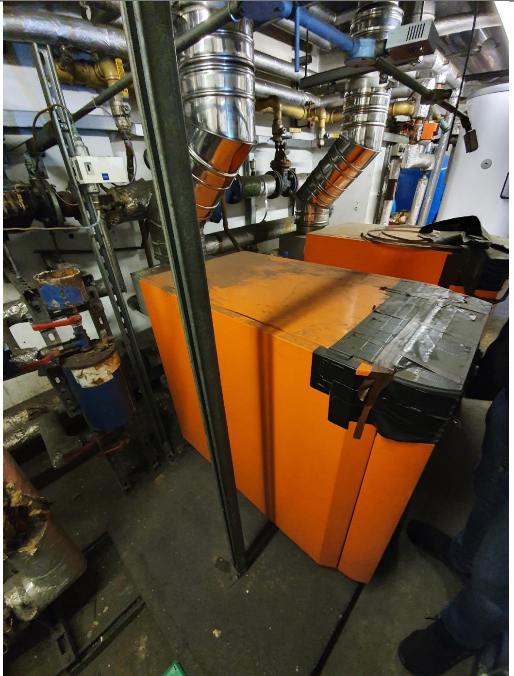
Boiler Room – Asbestos Debris to walls
